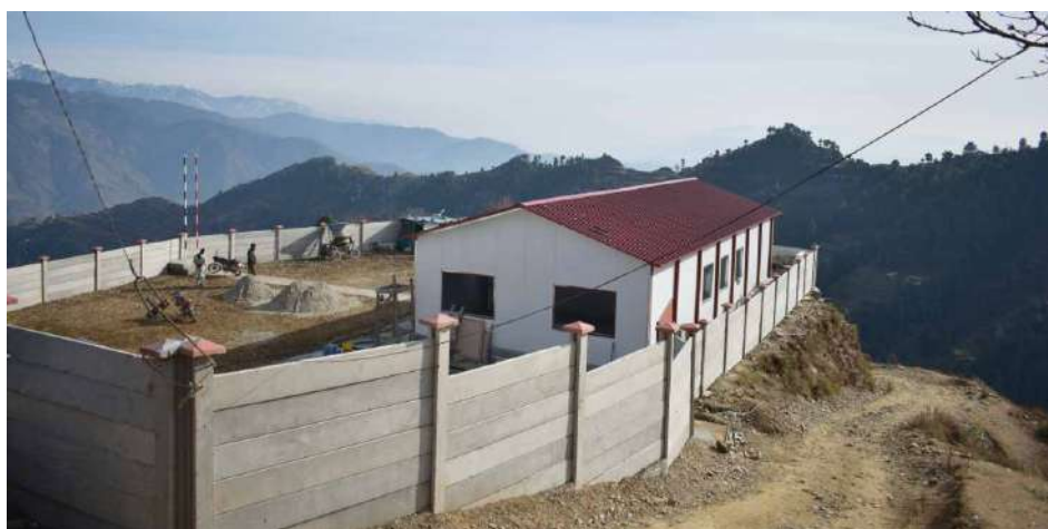
GPS Qazi Khait UC Bhogarmang Completed 89%
