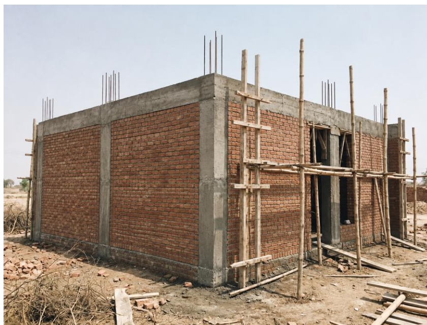
Figure 6.2 Confined masonry under construction: tie-columns cast against toothed panels with a continuous bond beam
