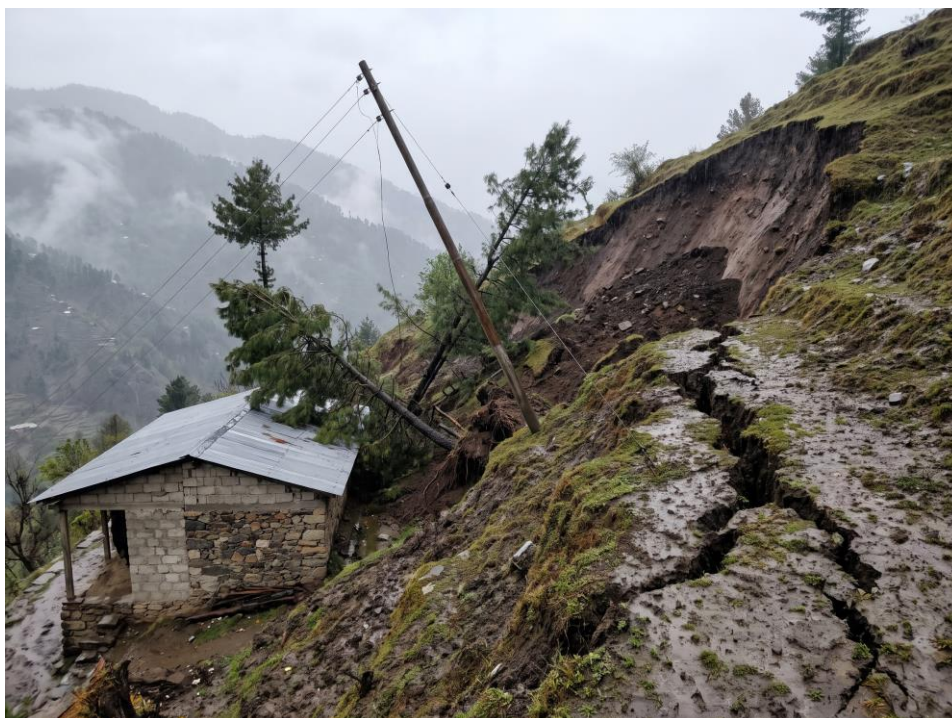
Figure 9.1 Head scarp and crest-parallel tension cracks above a building
