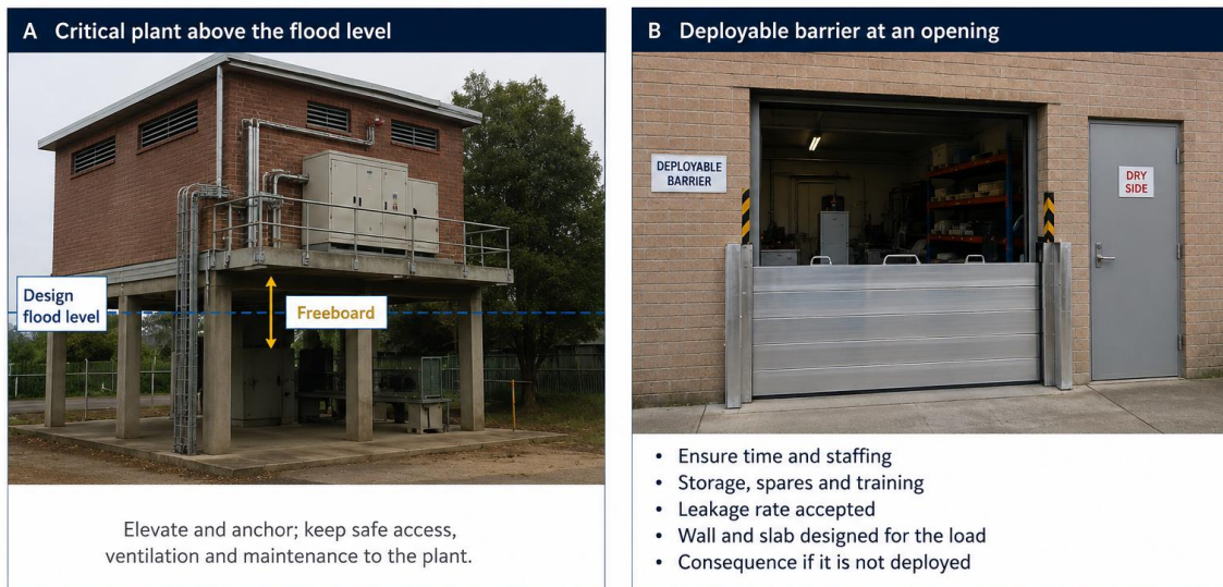
Figure 7.6 Elevated critical plant and a deployable barrier
