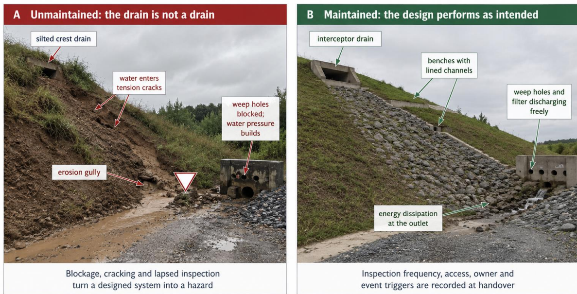
Figure 9.3 Slope drainage in maintained and unmaintained states
