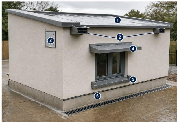
Figure 10.3 Water-shedding at the principal envelope interfaces
