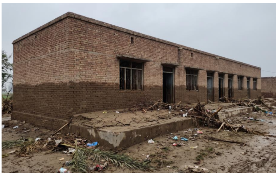
Figure 7.2 High-water mark after flood recession, one basis for the design flood level
