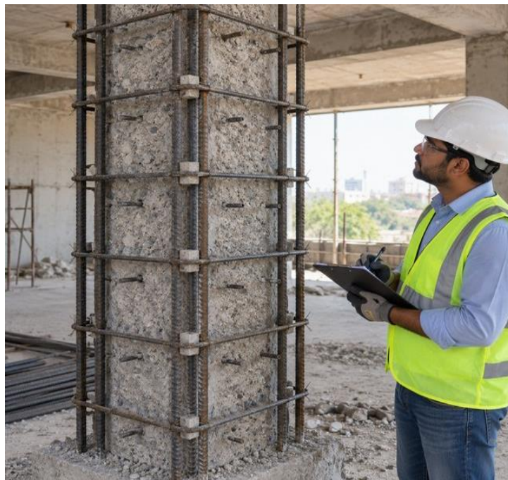
Figure 14.2 A column prepared for jacketing (illustrative, digitally generated; not a project record)
