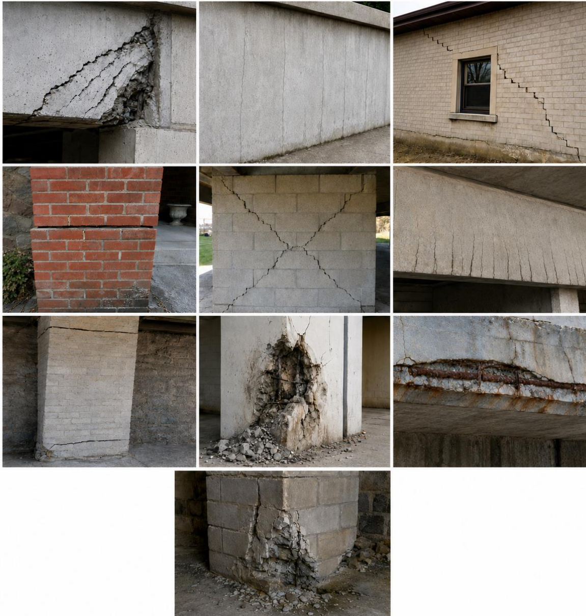
Figure 9.1 Crack mechanism patterns
